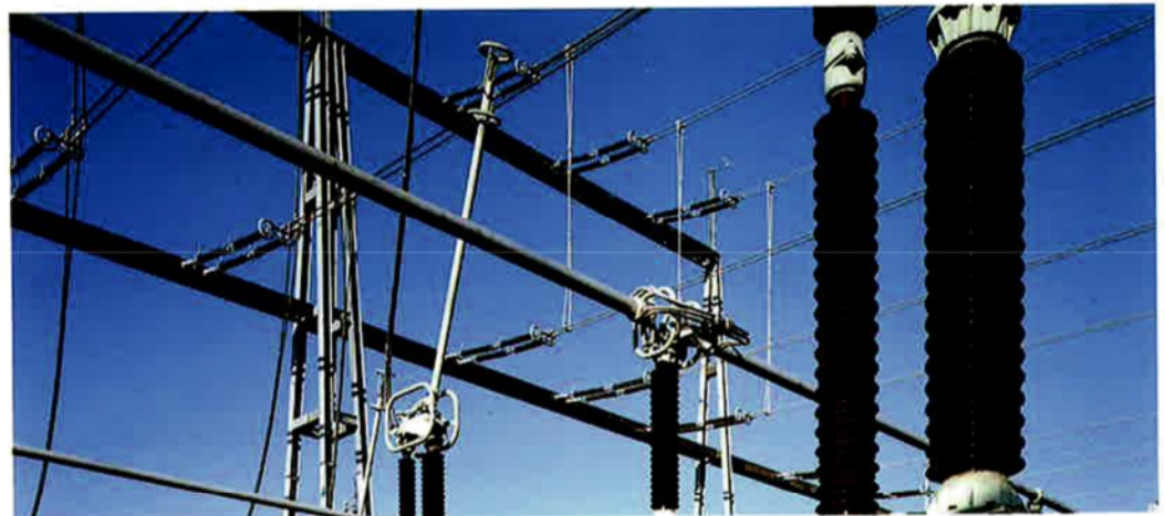
Tubular Busbar Substation
